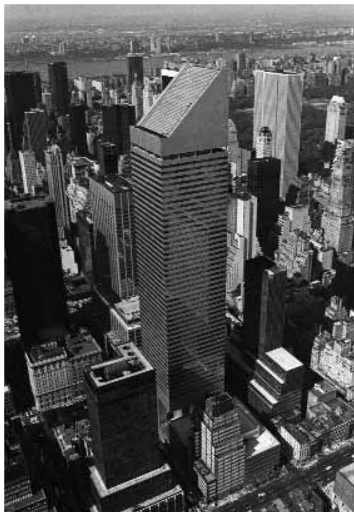
The Citicorp Center opened with an inadequate structure which could have failed in a severe storm. It was repaired at night over several months, unbeknownst to the building's occupants or people living in the neighborhood.
